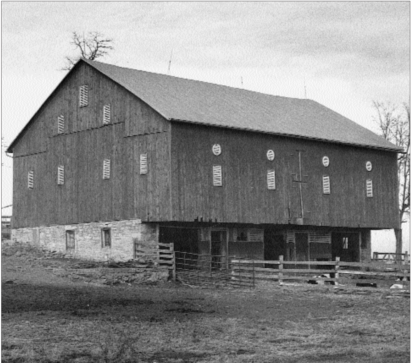
Fig. 1: This barn in Cumberland County, Pennsylvania, clearly depicts the forebay projecting over the barn's lower-level foundation.
