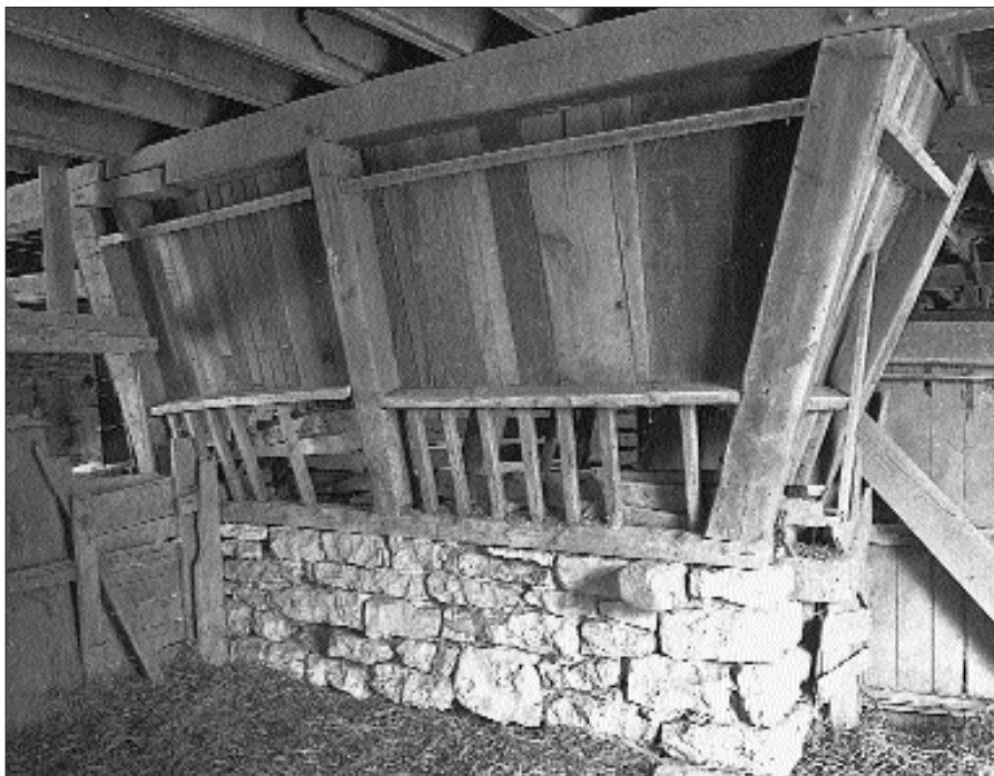
Fig. 13: Manger on lower level. This small section is all that remains of a manger that once ran almost the length of the barn.
